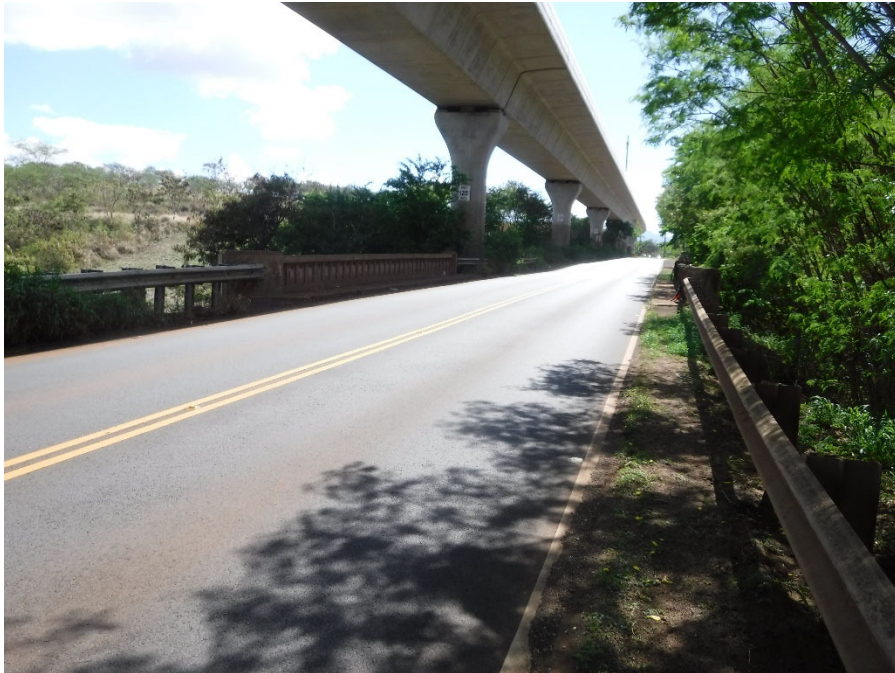
PHOTO 2 WEST APPROACH LOOKING EAST
