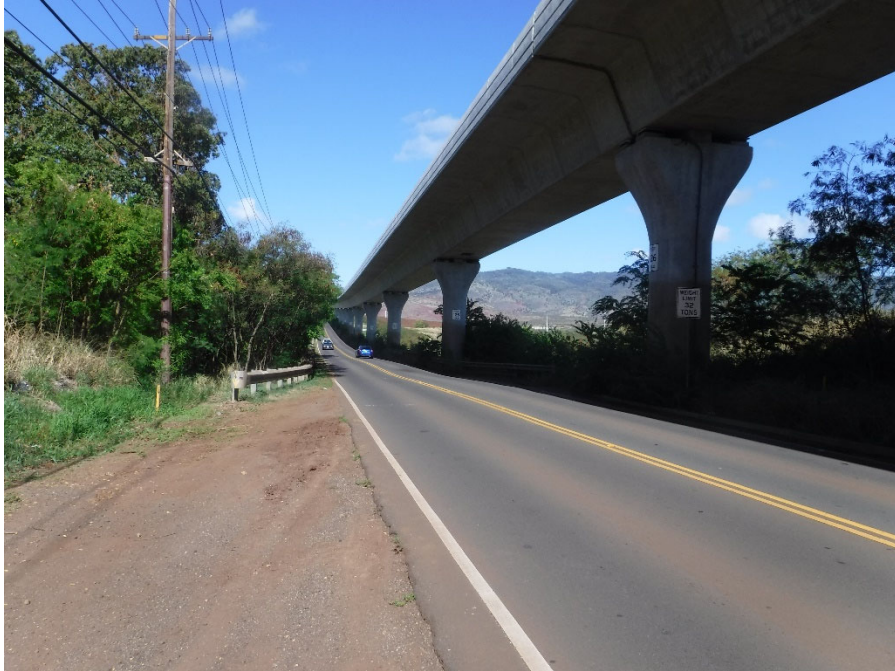
PHOTO 1 EAST APPROACH LOOKING WEST
